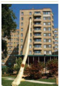
The advanced modular evacuation system is triggered by a fire alarm; the chute unfolds automatically from the structure. The user enters the chute through automatic doors and slides down, landing on a cushioned landing pad.
